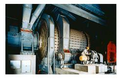
At the Dezhou Shandong Huaneng Power Development Co. Ltd. power plant in China, sealing air is used to contain hot exhaust air laden with coal dust in the neck of a coal mill. The ideal solution: An **Espey WD200/500**. Operating conditions: p = 1.08 bar (15.66 PSI); t = 110 °C (230 °F); n = 15.8 min<sup>-1</sup>.
